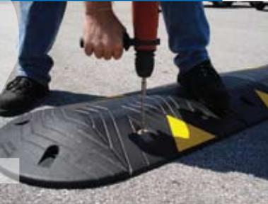
Beginning with the center piece, start drilling through the preformed holes in the module until you have reached a depth of four inches into the pavement.
