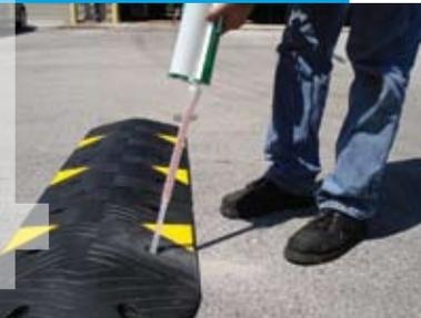
Place one complete pump of resin into each hole, keeping in mind that the resin will dry quickly.
